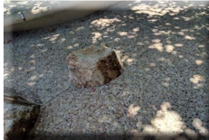
Aggregate Concrete With Boulders
