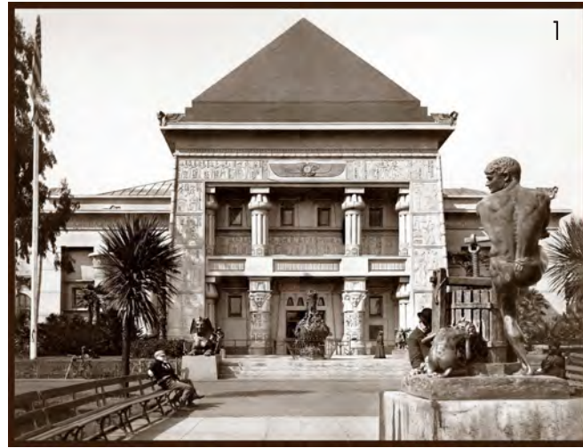
Original Egyptian Revival style Fine Arts building built in 1894
