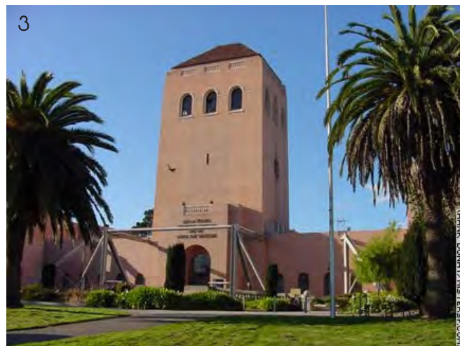
Temporary tower replacement post-earthquake in 1989
