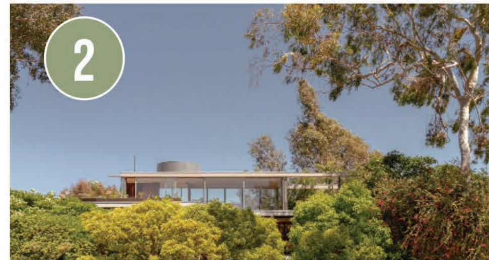
Neutra DVL Research House - Built in 1950 HCM - 1997
