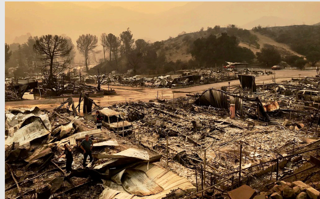
The upper lot of Seminole Springs mobile homes completely destroyed by the Woolsey Fire
