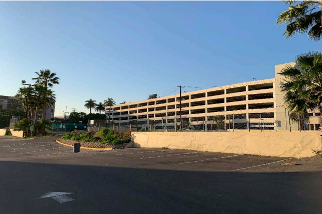
3 View towards the six level parking structure on Shatto St.
