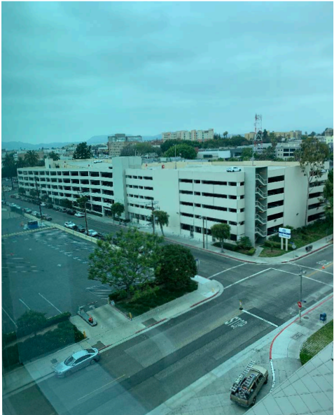
6 View of the site from the 6th floor of the Medical Pavilion South Tower
