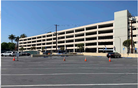
1 view of hospital parking structure
