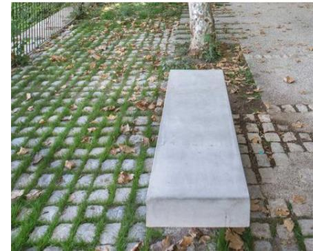
Street pavement detail - permeable paving
