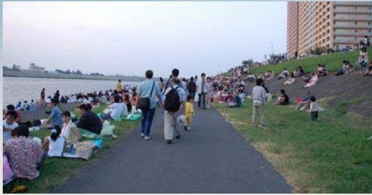
EARTHEN LEVEL WITH CONTINUOUS CREST OF 16.5 FEET ABOVE SEA LEVEL FOR FLOOD AND SEA LEVEL RISE PROTECTION
