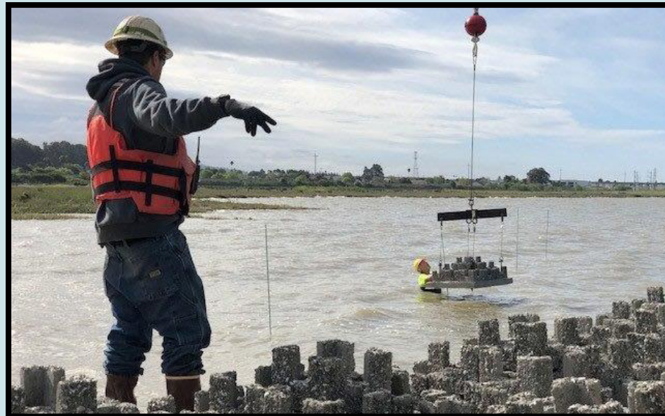
Reef Structures Being Testing at the Giant Marsh Project Richmond, CA
