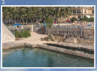
Pool deck has deteriorated and is collapsing into the ocean.
