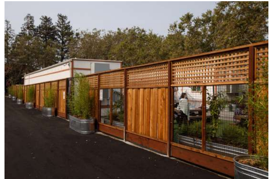
Fig. 54. Fremont Housing Navigation Center
