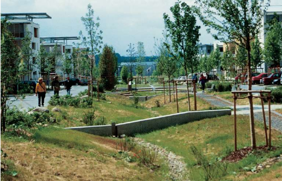
Fig. 48. Large bioswale with check dams
