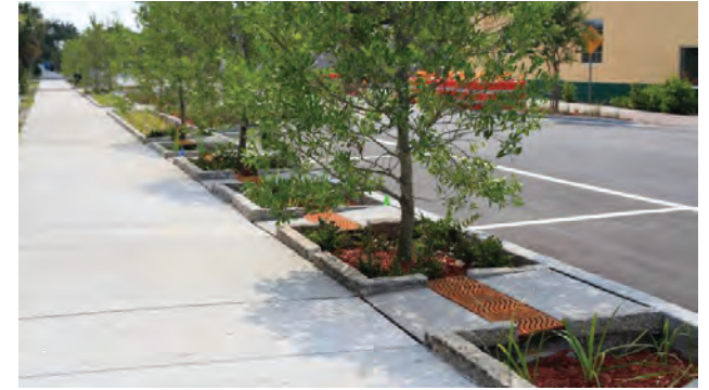
INTERCONNECTED TREE WELLS & SWALE: With energy dissipation weirs and grasses.
