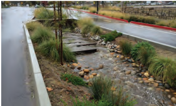
MEDIAN BIOSWALE: With energy dissipation weirs and grasses.
