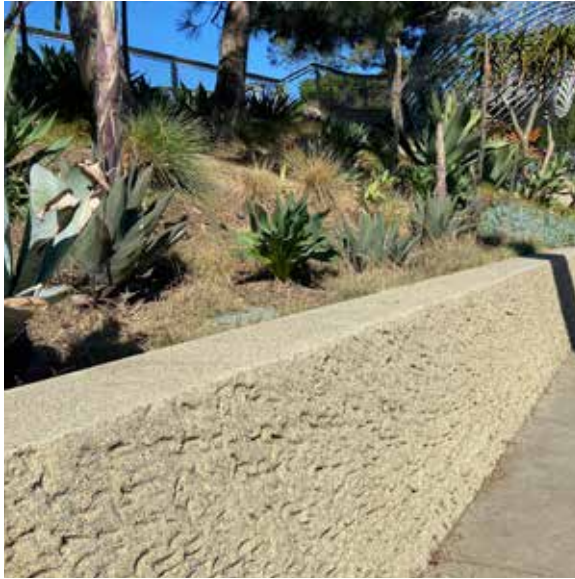
CONCRETE AND STONE Textured retaining wall
