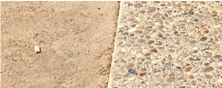
DECOMPOSED GRANIT AND CONCRETE WITH SMALL AGGREGATE
