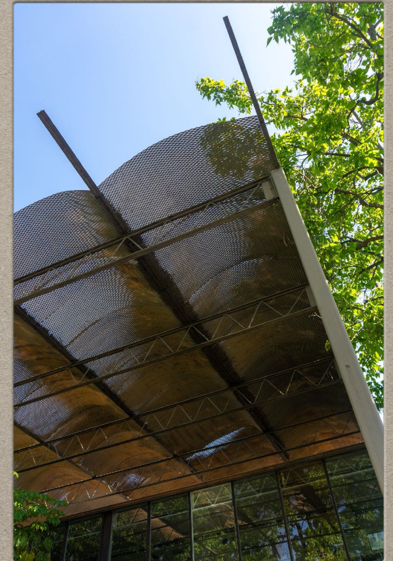
Detail of aluminum mesh shade from north side main entrance
