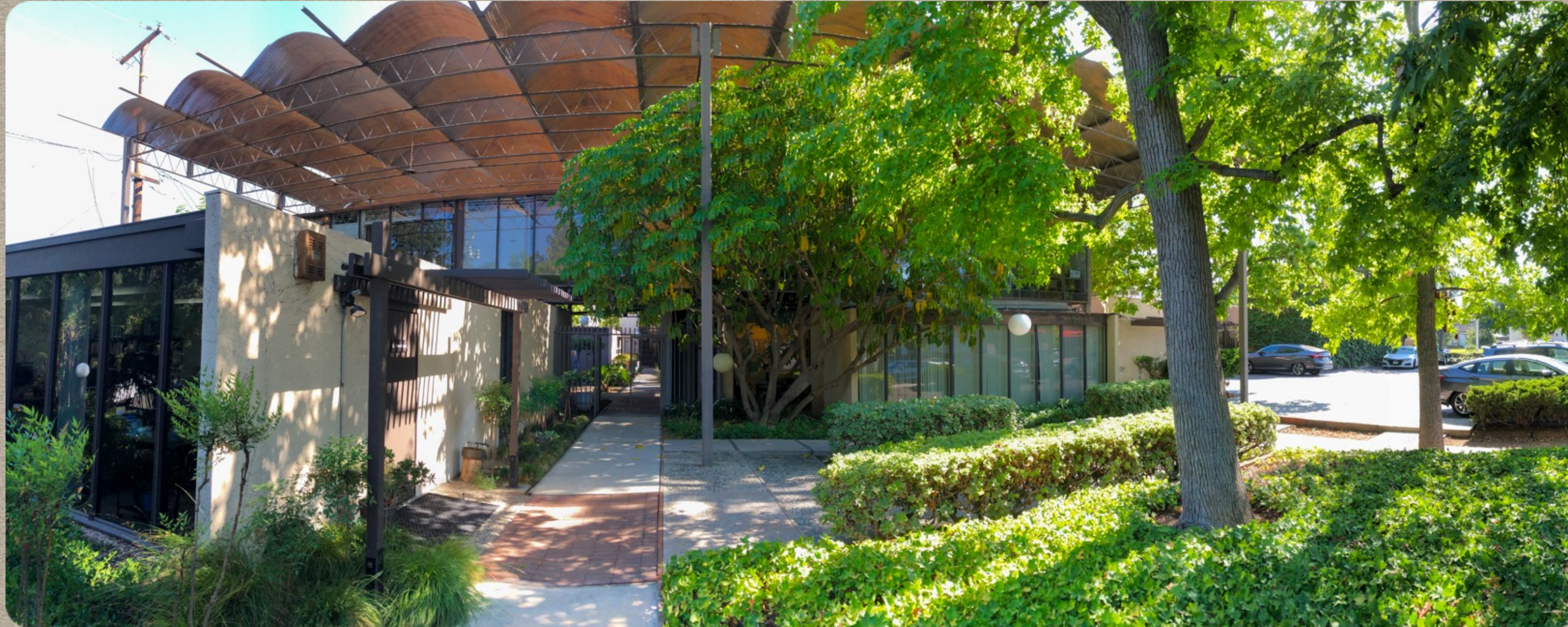
Today's view of main entrance looking south
