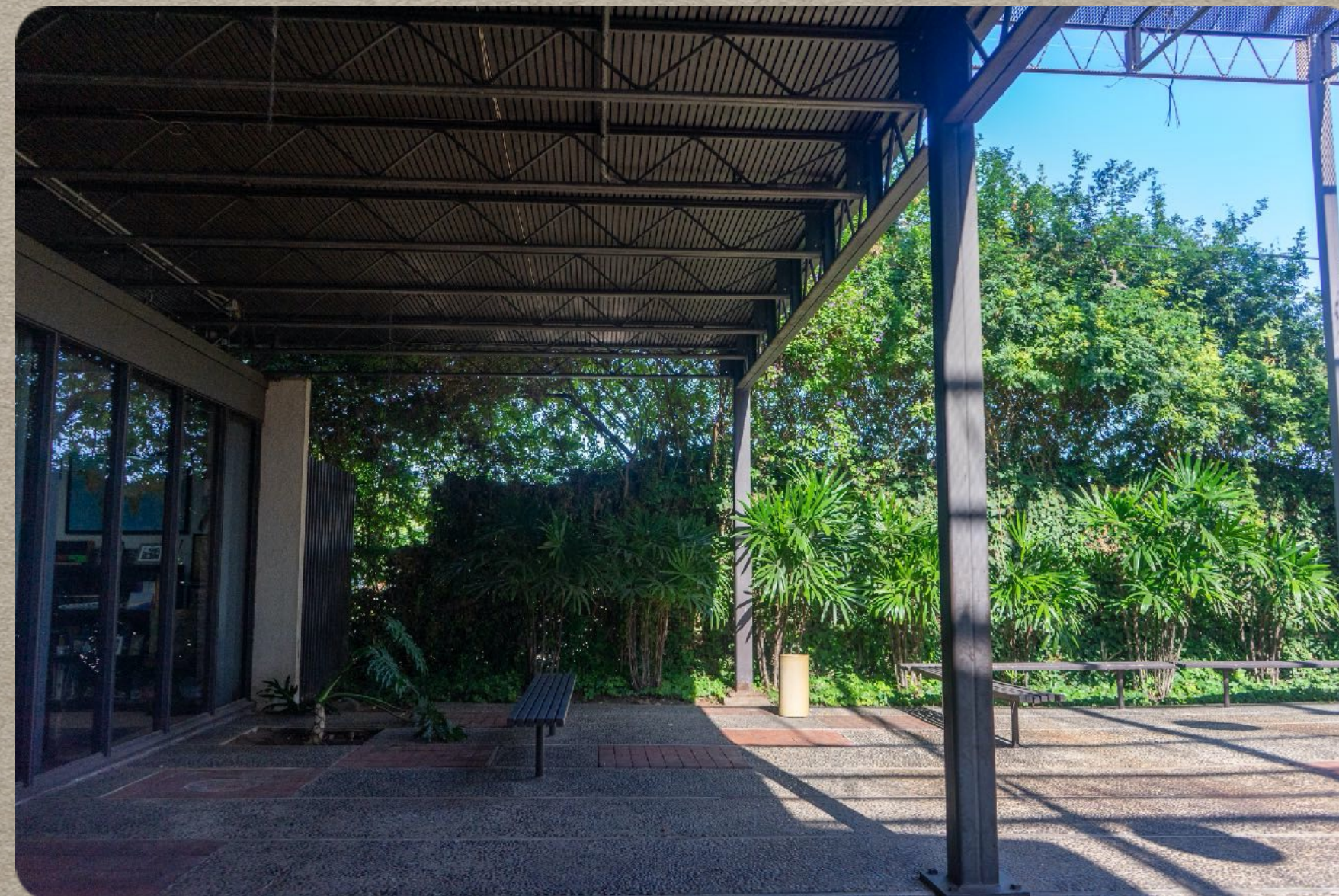
Second floor steel post and beam construction
