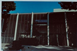
ENTRANCE SCREEN & DOORS - SCULPTURE
