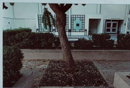
GIRDLED TREE TRUNK BY METAL GUARD
