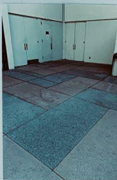
NE CORNER, DOORS & CONCRETE
