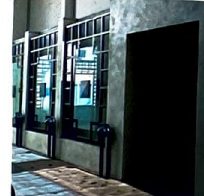
VESTIBULE ADJACENT TO FREUD PLAYHOUSE. APPROX 9' HIGH. ADOPTED AS PART OF 1990s RENOVATION.
