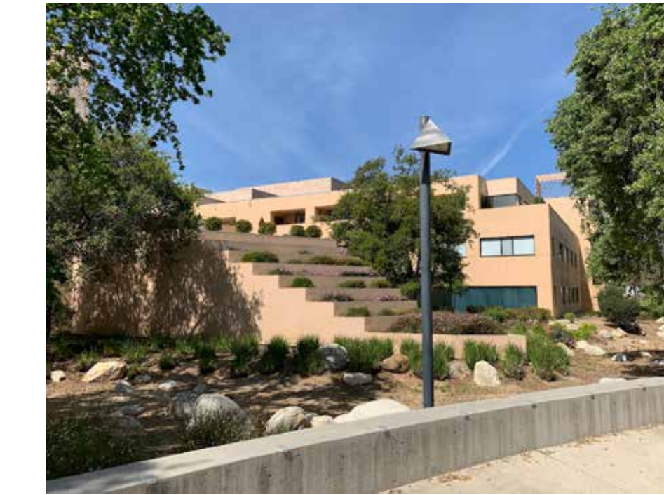
No Front Entrance.
