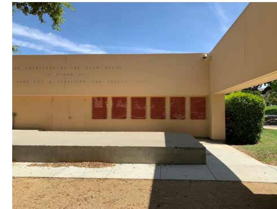
Underutilized Stage. Planned as an Amphitheater this space doesn't work.
