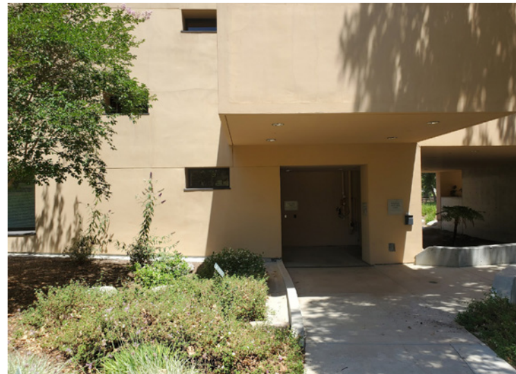
⑤ Hidden stair entrance to the second floor terrace
