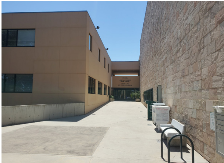
④ Hidden entrance to City Hall
