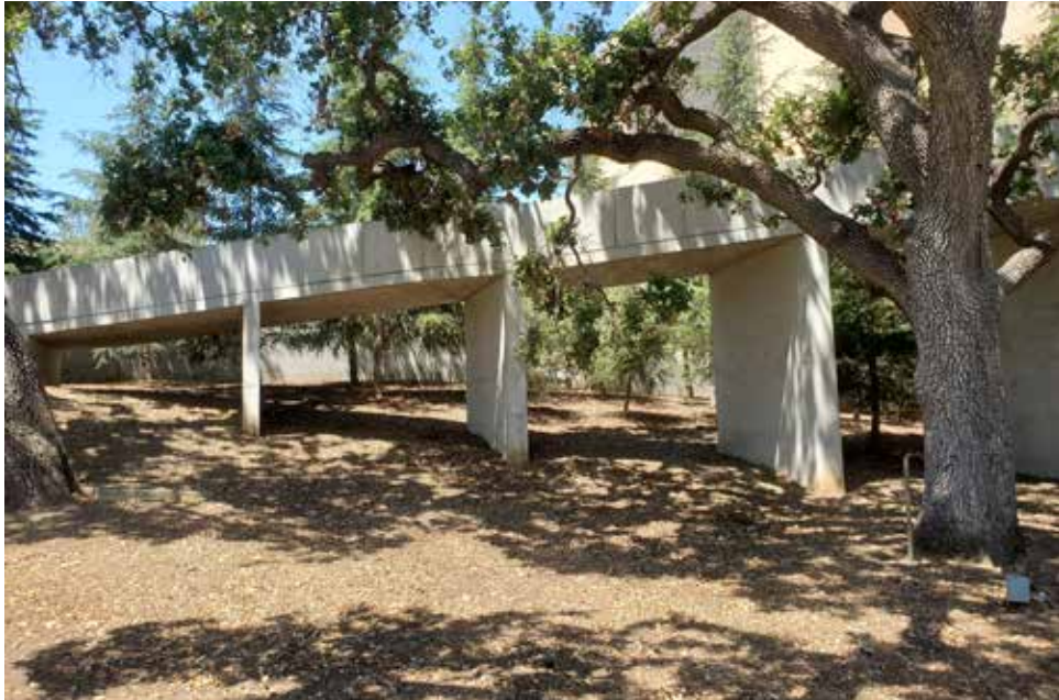
Pedestrian ramp to 3rd floor of building
