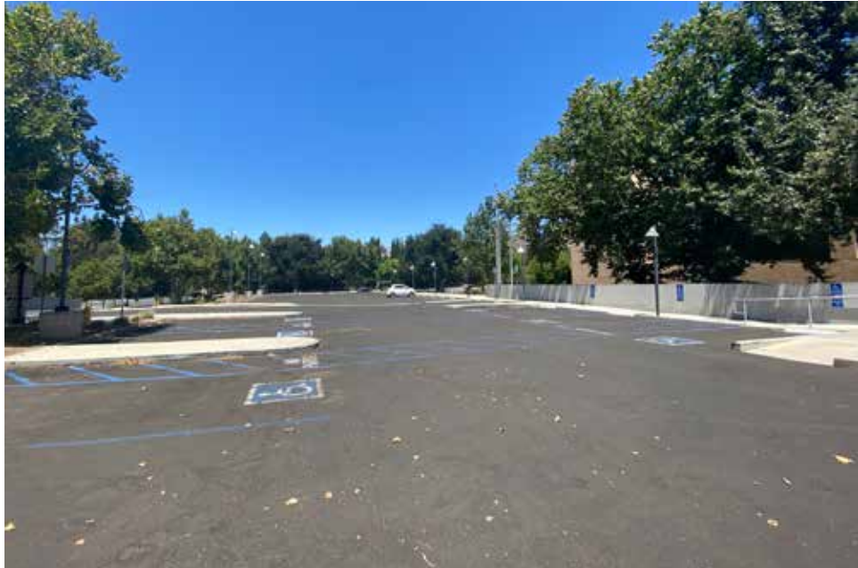
Parking lot at the intersection of Thousand Oaks Blvd and Dallas Dr.
