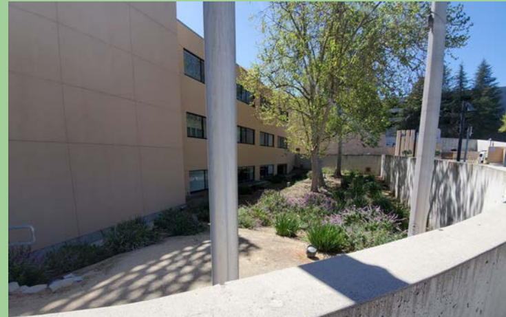
2 Lower grade: entrance is on the second level, but there are first-floor windows near the entrance
