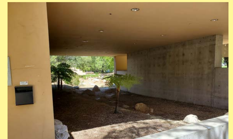
6 Tunnel: area underneath is heavily shaded
