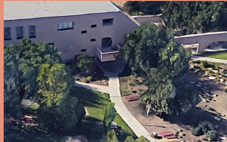
10 Stairwell: building entrance with a second-floor balcony
