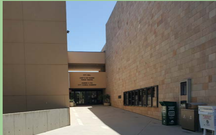
1 Existing main entry: tucked away and not very prominent
