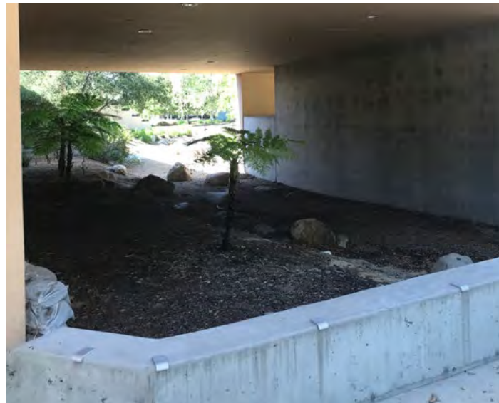
Picture 4: Hidden shady area under building structure.
