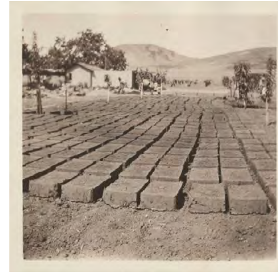
PHOTOGRAPH OF THE ADOBE BRICKS THAT WERE MADE FOR THE CASA CONEJO IN 1922. SOURCE: calisphere.org
