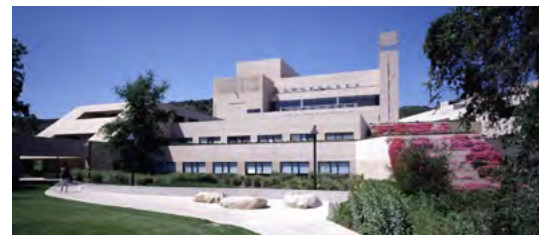
① SITE - CIVIC ARTS PLAZA Source: foursquare.com
