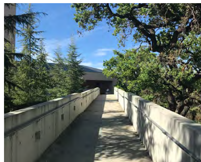
Picture 6: Bridge/ramp access to building at Level 3. Tree canopy walk.
