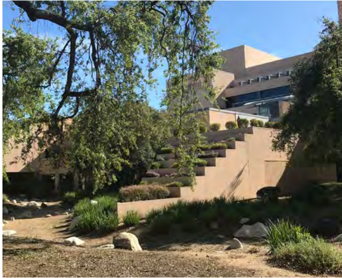
PICTURE 7: Stepped planter. Potential stair access to Level 2.
