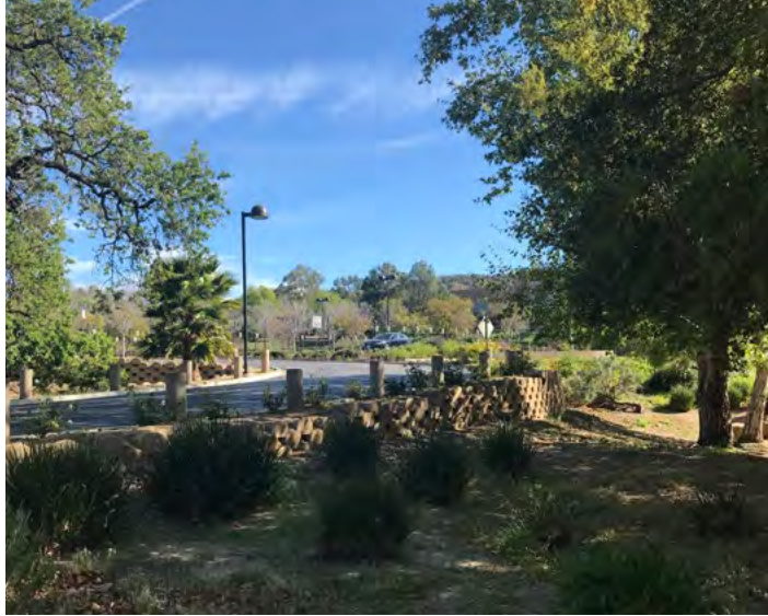
PICTURE 1: The Lakes Dr. edge. Retaining wall + slope.
