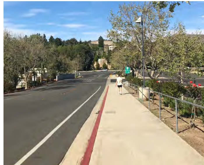
PICTURE 6: Dallas Dr. Sloped street. Access to parking and loading dock.
