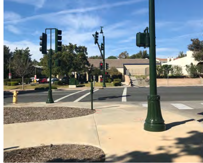
PICTURE 3: Thousand Oaks Blvd. @ Lakes Dr. Open, flat area.
