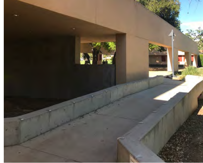
PICTURE 3: Concrete path/bridge with thick low walls. Disconnected from landscaped areas.
