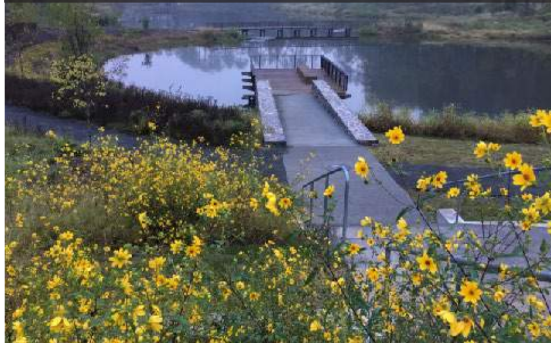
02 AFTER- RECLAMATION POND
