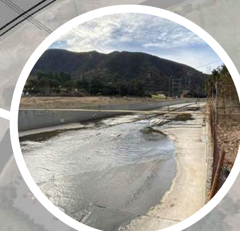
5) PEEL BACK THE CONCRETE OF THE LA RIVER
