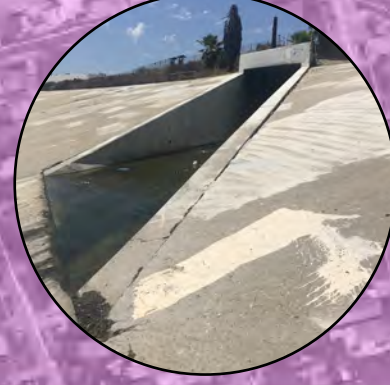
CONCRETE RIVER SIDES AND STORM DRAIN OUTLETS
