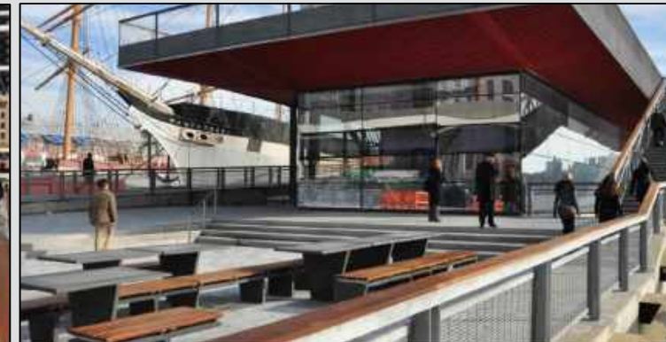
roof garden on pier 15
