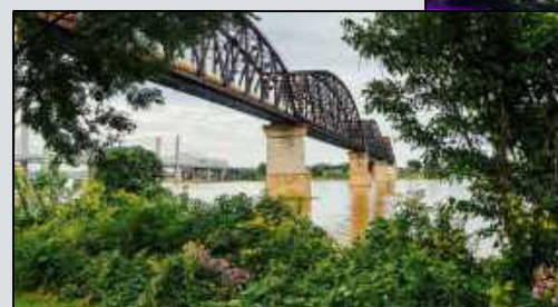
big four bridge
