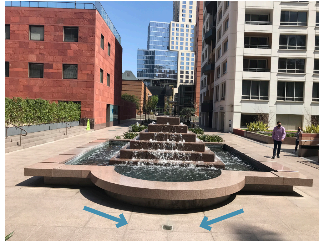
Connecting Walks Built on Structure and Served by Area Drains
