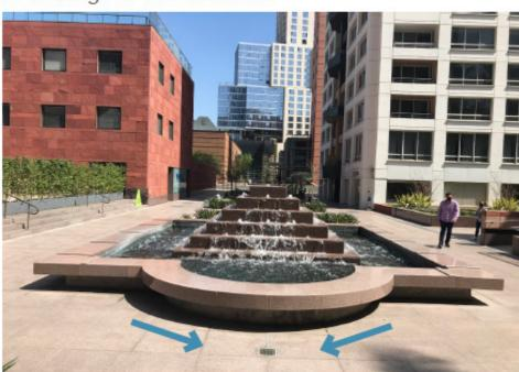
Connecting Walks Built on Structure and Served by Area Drains
