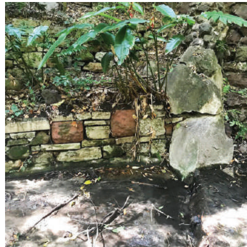
Dry stacked stone with larger stones to right.
