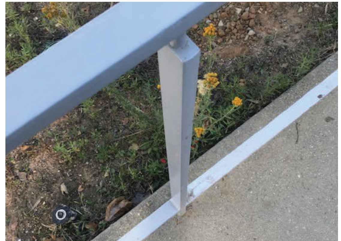
Detail of post connection on rail
