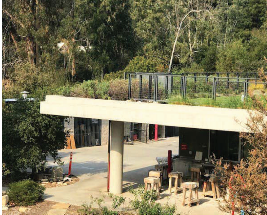
2nd floor roof garden and column with drain
