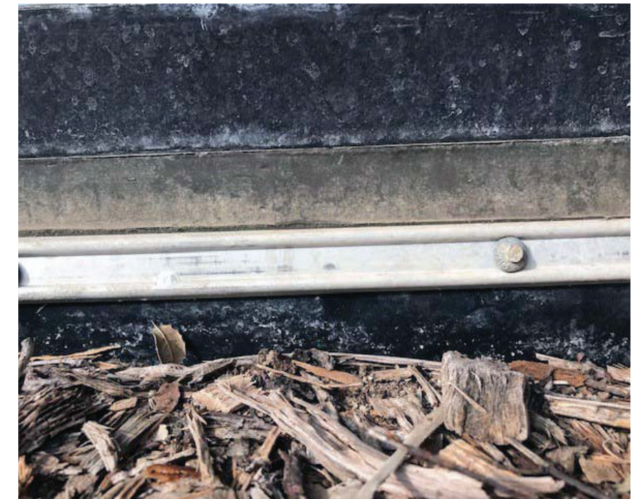
Flashing detail root barrier (black) also visible
