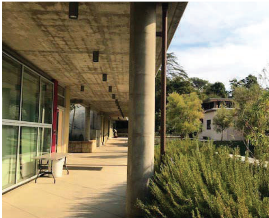
Column close up with drainage
