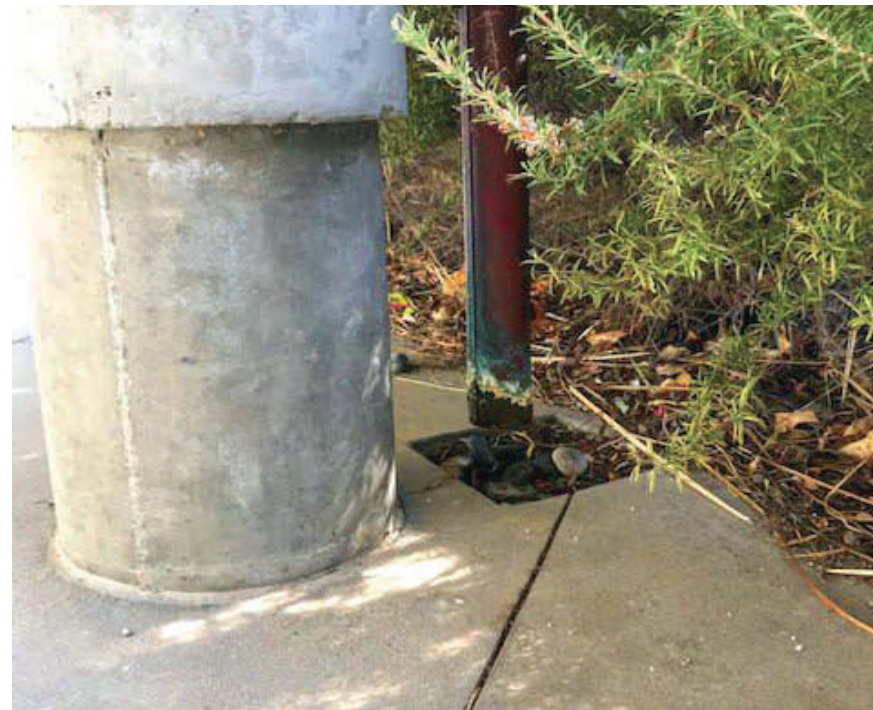
Close up of drainage into catch basin
