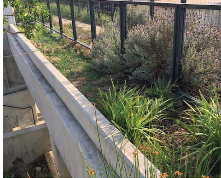
Close up of 2nd floor roof garden edge
