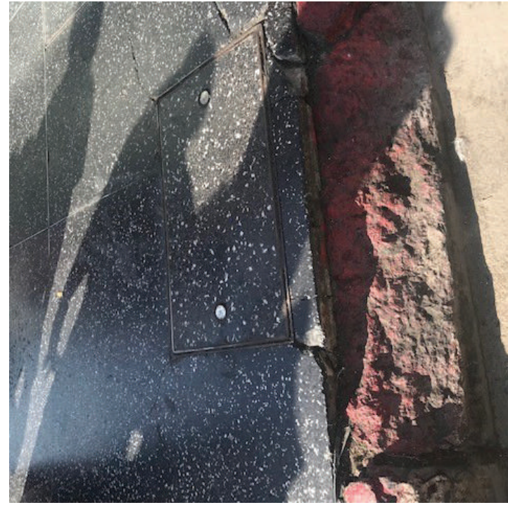
Broken curb interface with terrazzo pavement. Broken divider.
