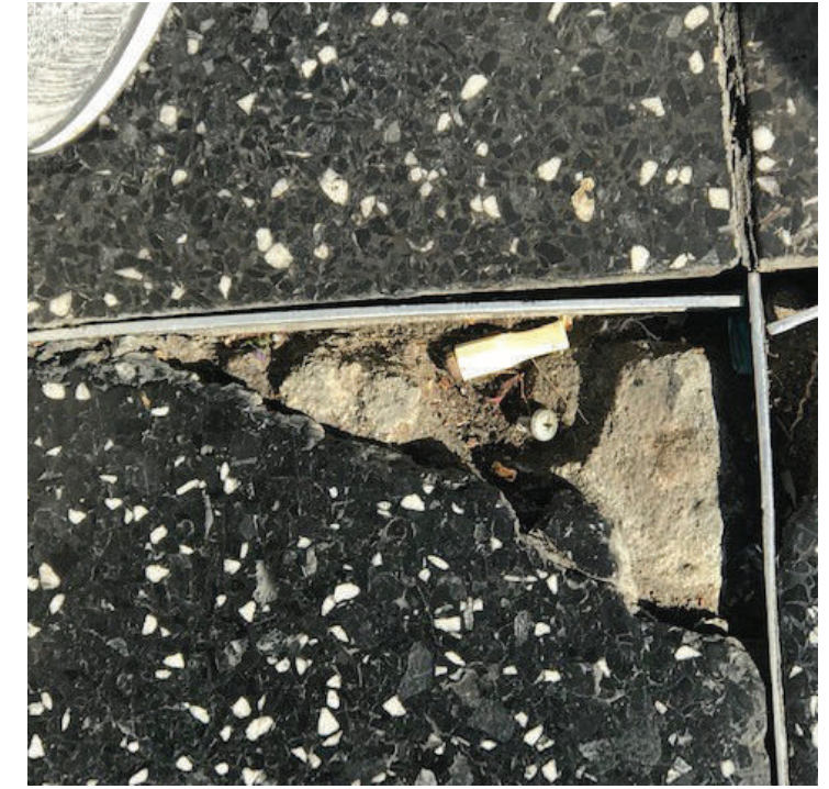
Detail of broken terrazzo and warped dividers.
