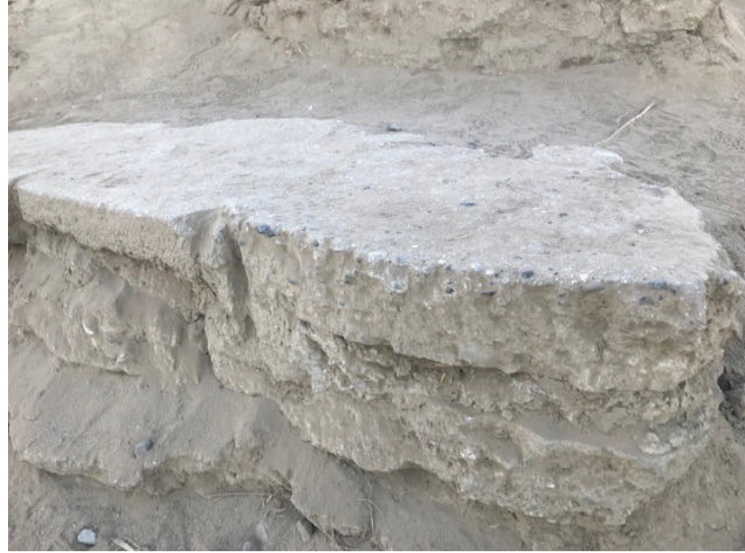
Stair detail 4-6 layers of 2" broken sidewalk
