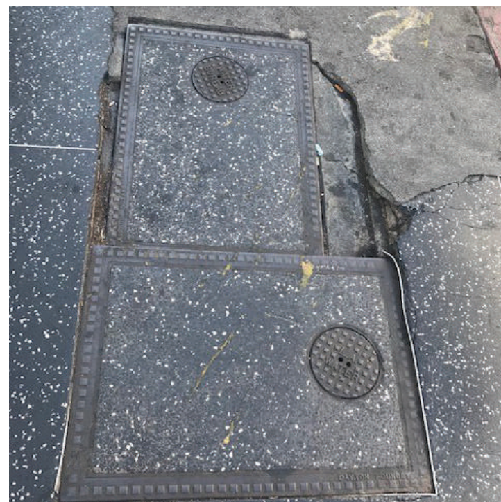
Utility Box covers
