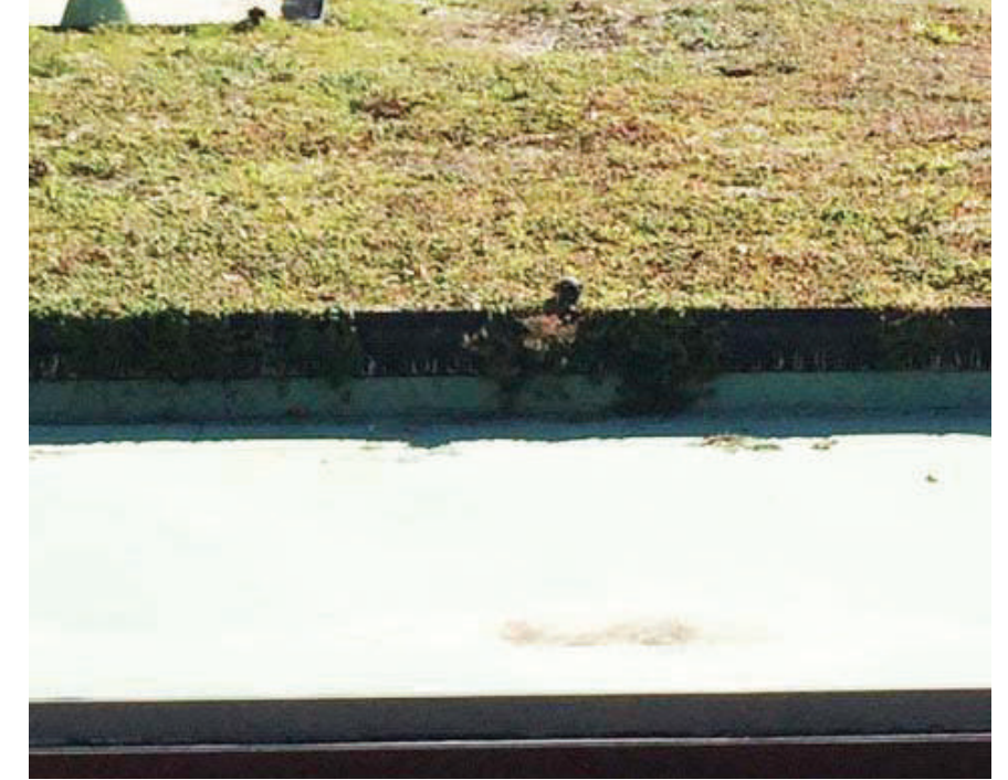
Close up of Winter Hall intensive garden The draining layer is visible above the root barrier and elastomeric moisture barrier
