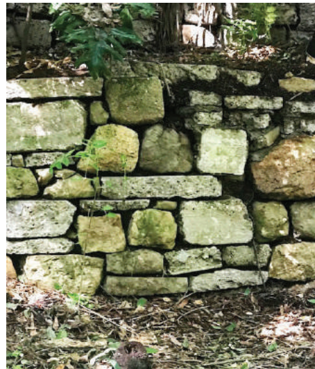
Original Dry stack stone wall with portions of broken sidewalk within original wall and above.
