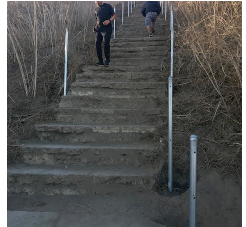
New railing being installed
