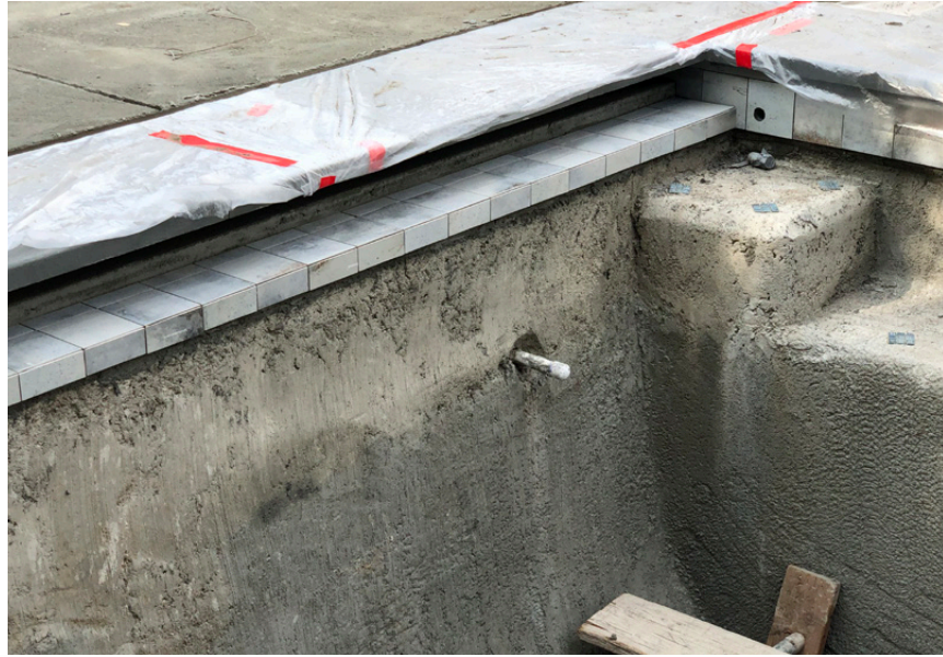
15. Close up of pool coping and autocover during construction
