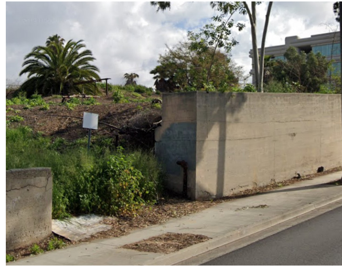
P1. West side condition of retaining wall
