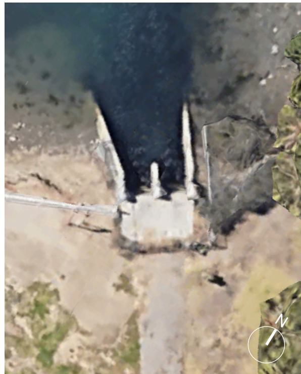
I1. Aerial image of the box culvert
