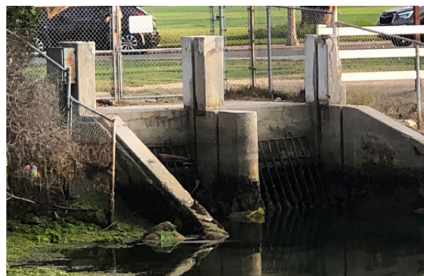
P7. Box culvert connection to Alamitos Bay
