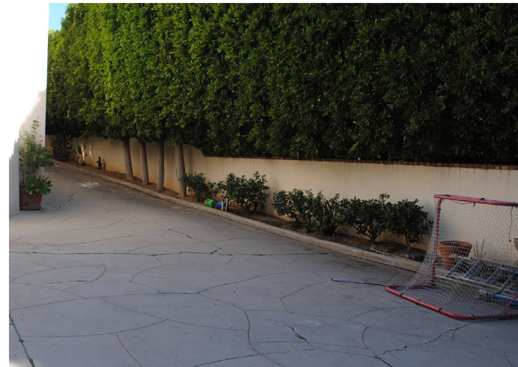
I2. View of side yard entry to rear yard
