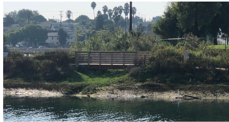
P4. View of walking trail bridge
