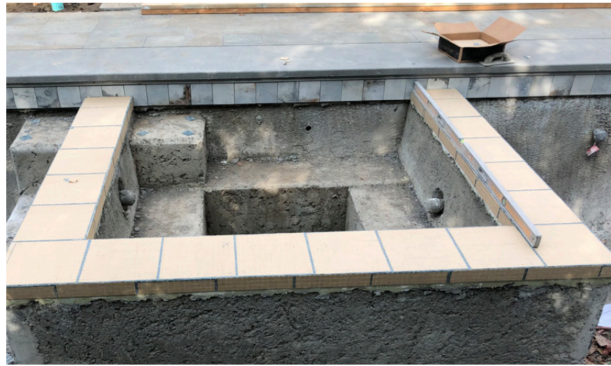
I4. Spa during construction
