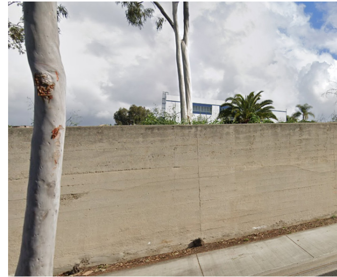
P2. Poured-in-place concrete wall
