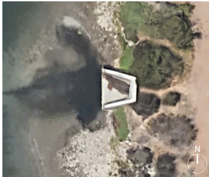
I2. Aerial image of pipe culvert
