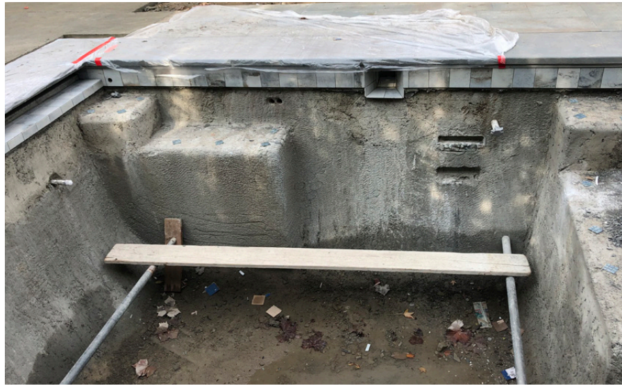
I4. Pool during construction
