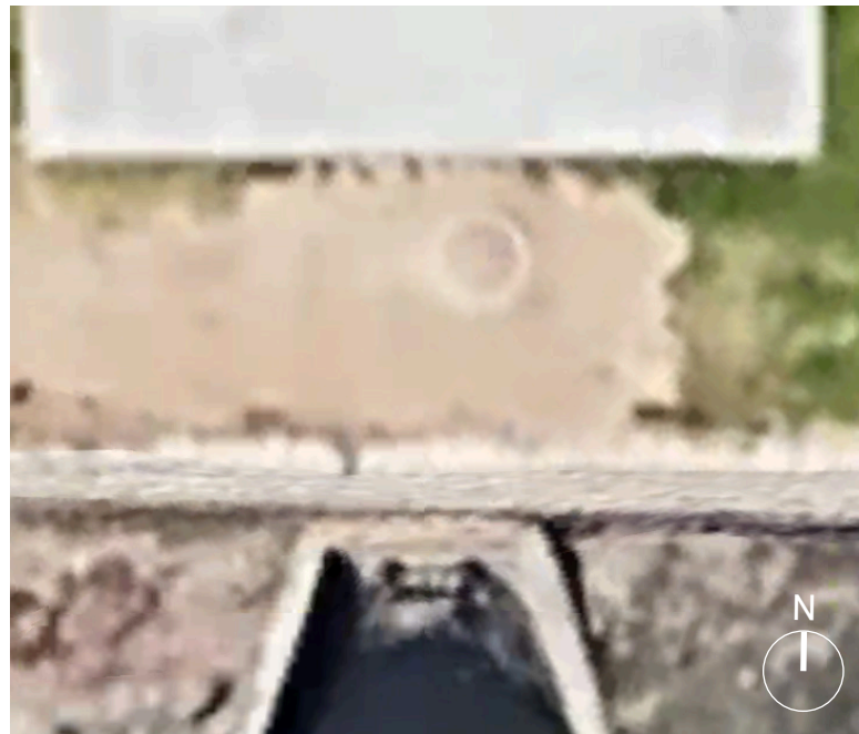
I3. Aerial view of manhole on grade above a pipe culvert
