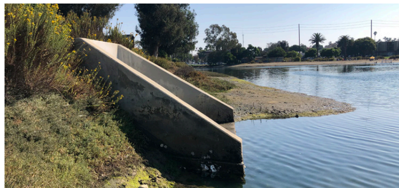
P8. Pipe culvert
