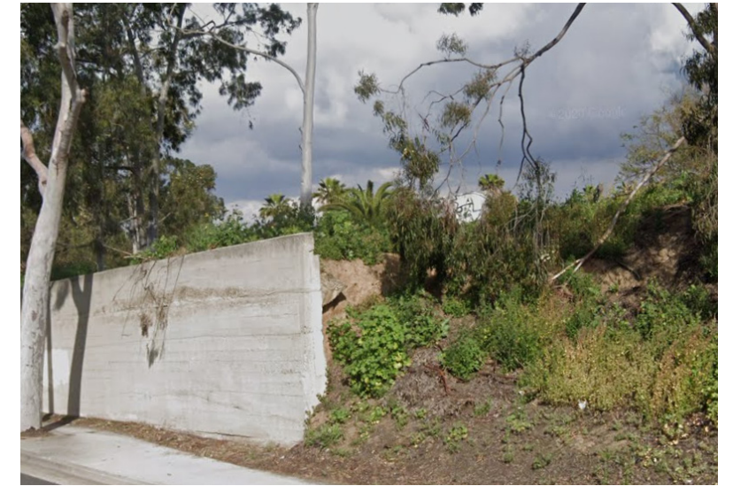
P3. East side condition of retaining wall
