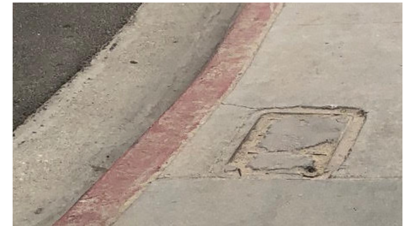
P3. Concrete curb and sidewalk paving
