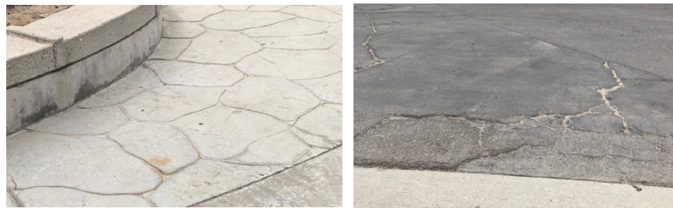
P1. Concrete with irregular paving design P2. Asphalt of parking lot
