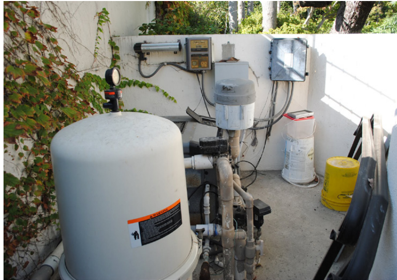
16. Image of the pool equipment
