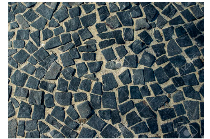
P6. Tile pieces with grout joint
