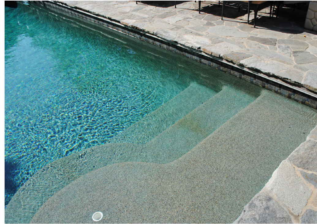
I1. Residence's old pool with baja shelf and steps
