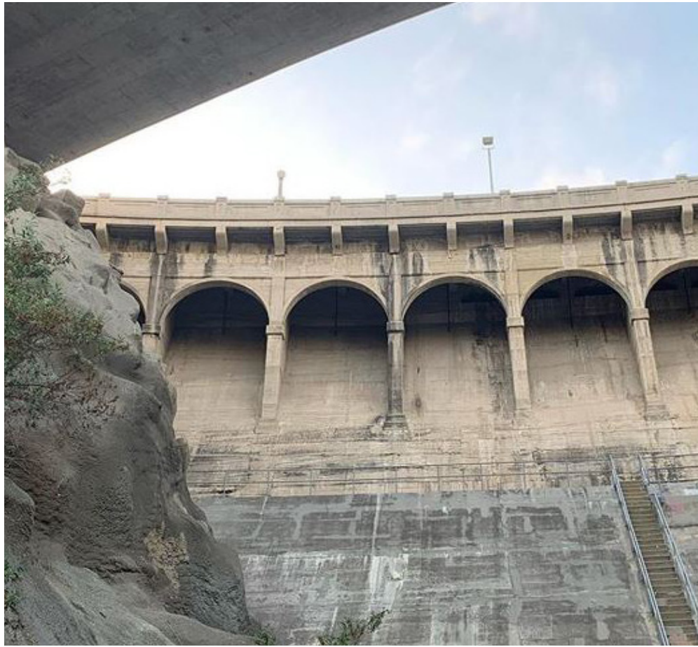
Devil's Gate Dam
