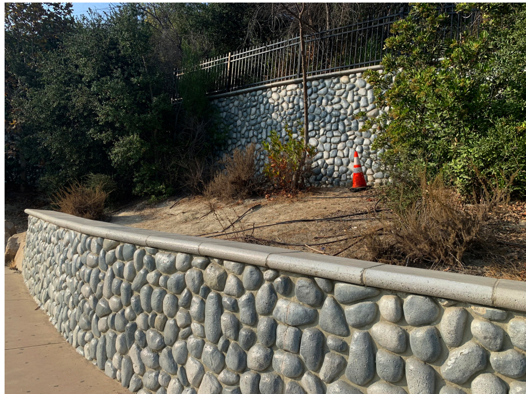
① Double retaining walls, the first 3.5' and the second 8'
