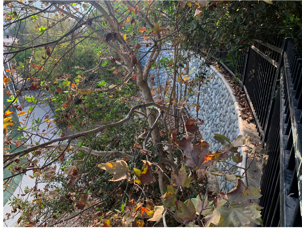
② View from above the top wall, along the fence
