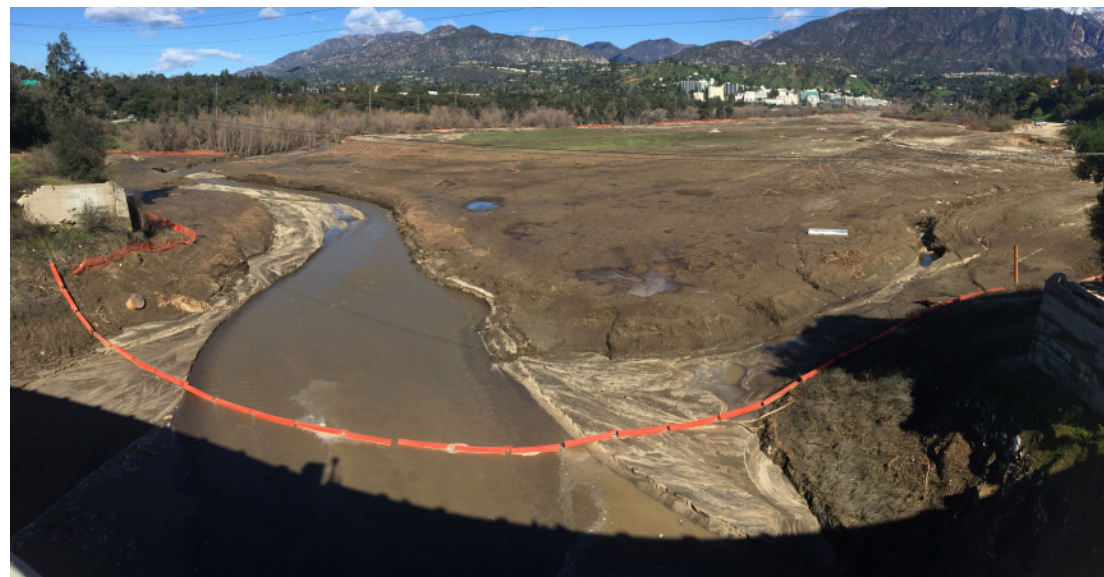
P3- The Hahamongna flood basin currently being dredged to improve the flood channel
