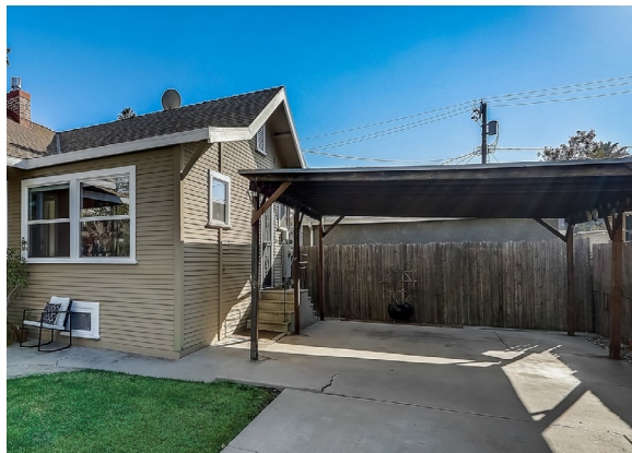
(P11) Carport with wood fence, side door into kitchen
