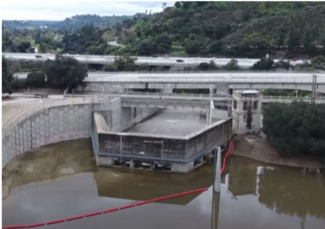
P2- The spillway filling after a rain event
