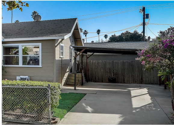
B (P10) Concrete driveway into carport
