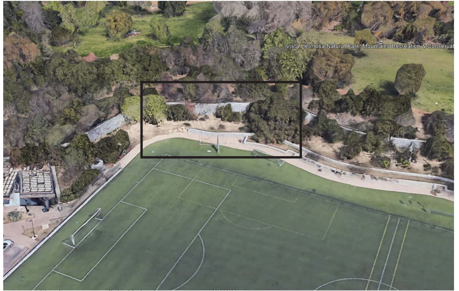
Soccer Field with retaining walls highlighted
