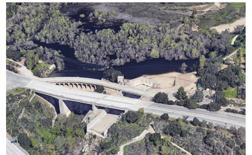
C. Devil's Gate Dam Area
