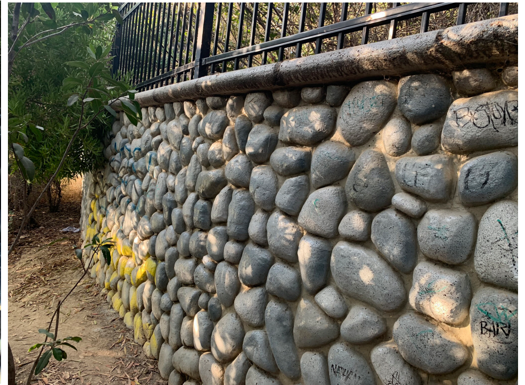
③ Close up of stone veneer retaining wall
