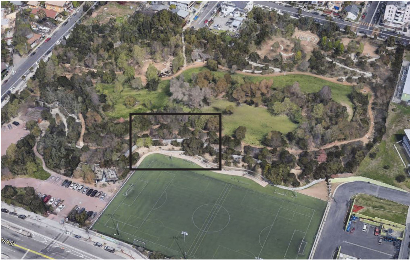
Vista Hermosa Park and Soccer Field, with retaining walls highlighted
