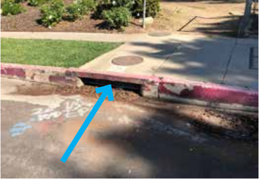
B. Typical Storm Drain
