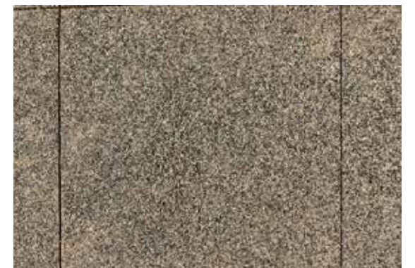
Exposed Aggregate on Conc. Structure
