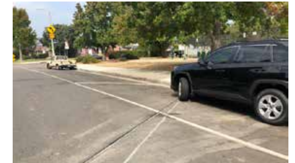
Ⓐ Road Cut for Diversion Weir
