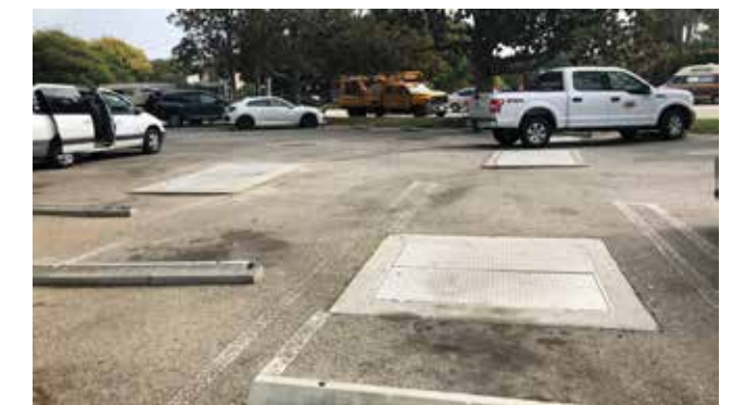
Manhole access for maintenance under the West parking lot of Mar Vista Park
