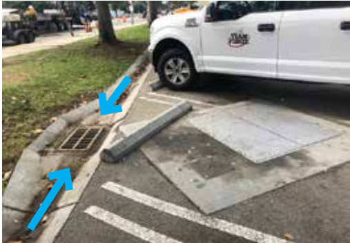
D. Catch Basin
