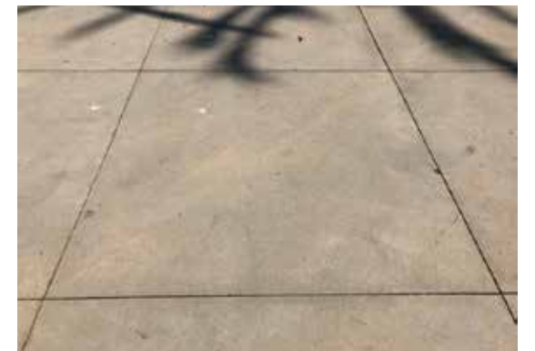
Poured Conc. on Conc. Structure
