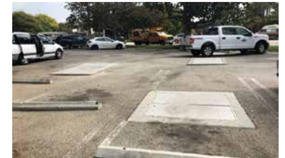
Ⓑ Manholes to Access Storm Vault, Flow Meters, Baffle Box, and Isolation Vault + Valve
