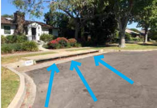
A. Entrance to Channel
