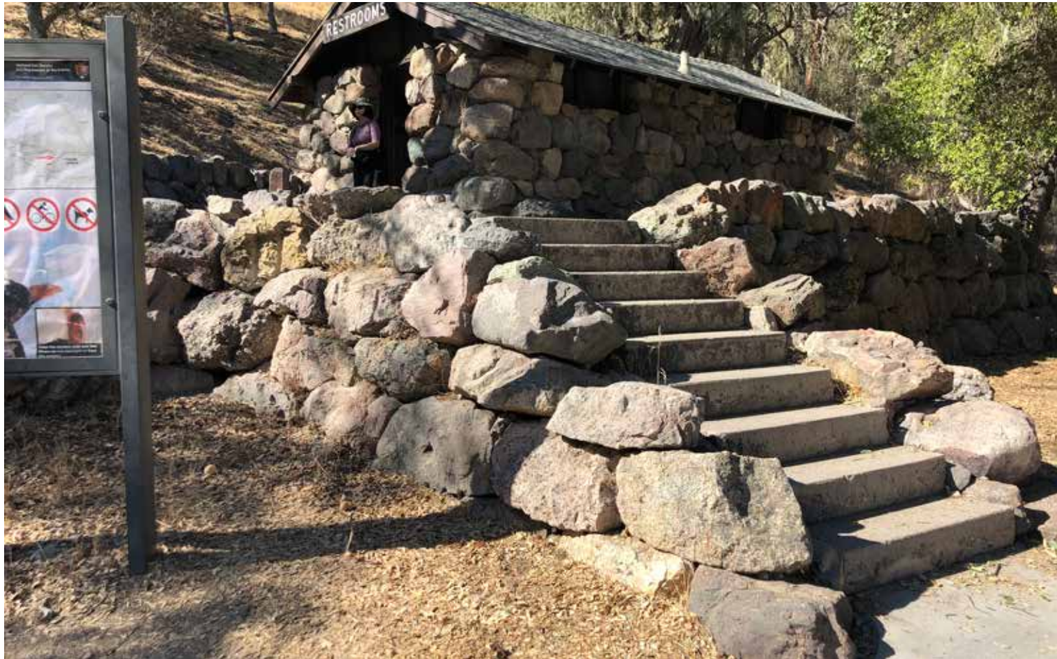
Looking West from Stair Base
