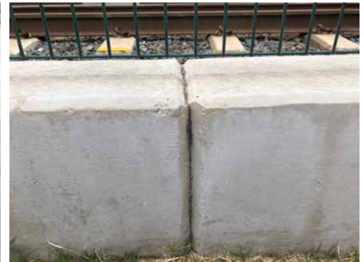
Concrete Expansion Joint
