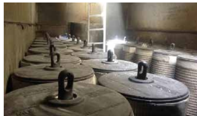
StormFilter cartridges inside the vault
