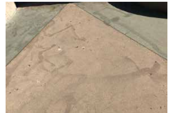
Colored Conc. on Concrete Structure
