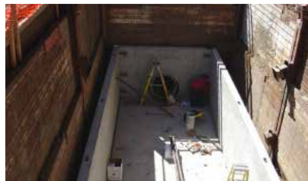
Submerged StormFilter Vault during construction of the channel
