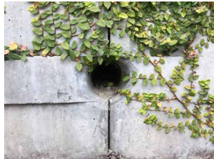
4" Weep Hole in Panel
