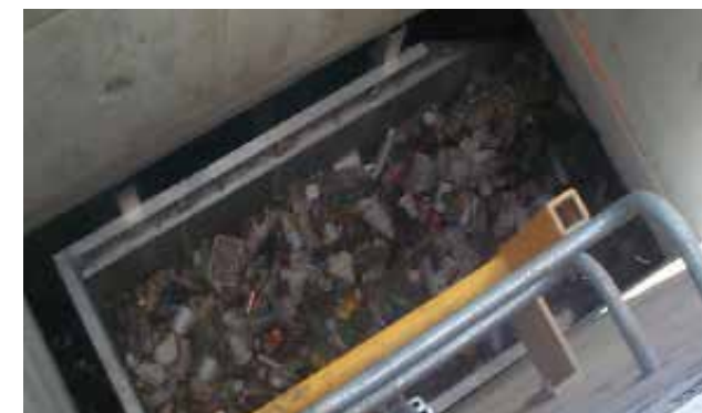
Baffle Box opened for debris removal
