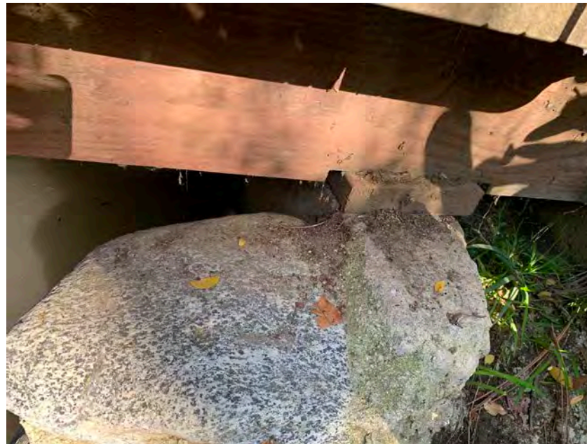
Beam on top of concrete base and on top joists and decking.
