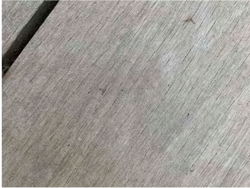
Decking and spacing.
