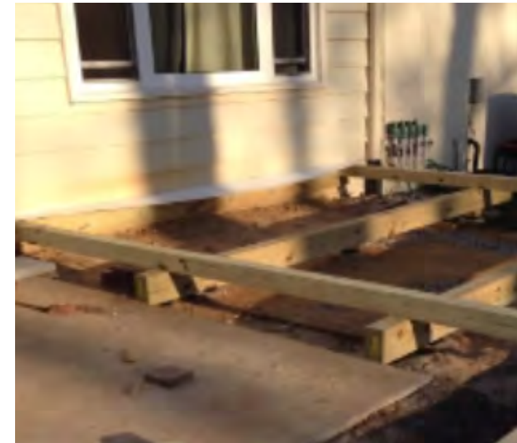
Ledger board used to attach deck framing and the house.
