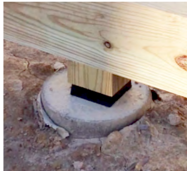
Cement footing with composite on top, wooden post and beam.
