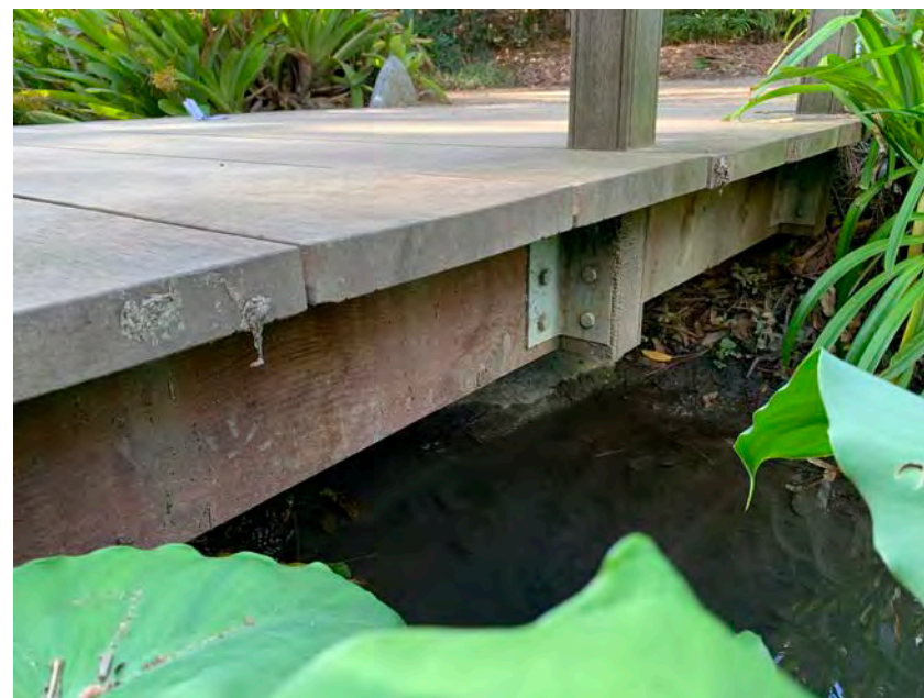
Joists with guard rails bolted in.
