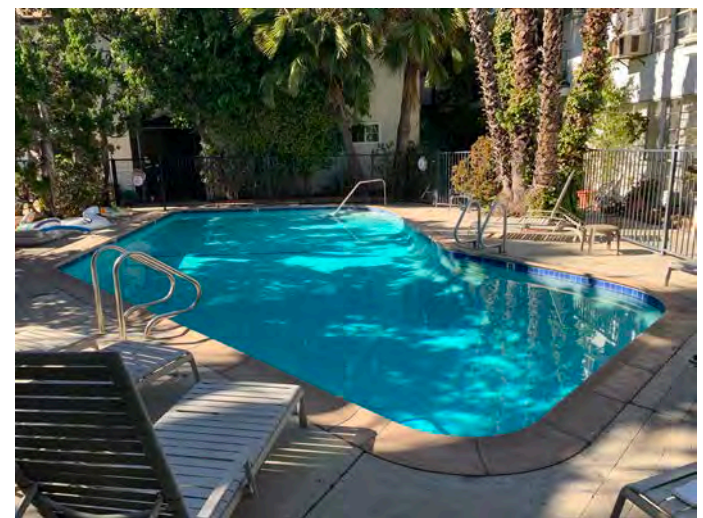
C. East side of the pool and in the back the west side of the pool and building entrance.
