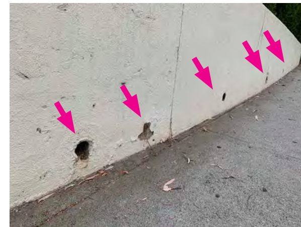
Drain holes along the north side of the retaining wall
