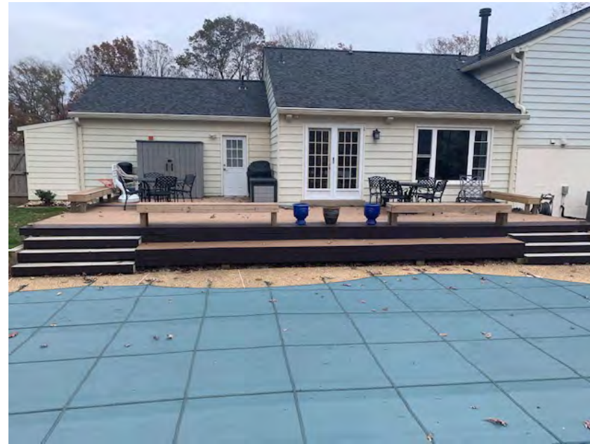
Front - facing west. There are two set of steps on each side and a long bench in between.
