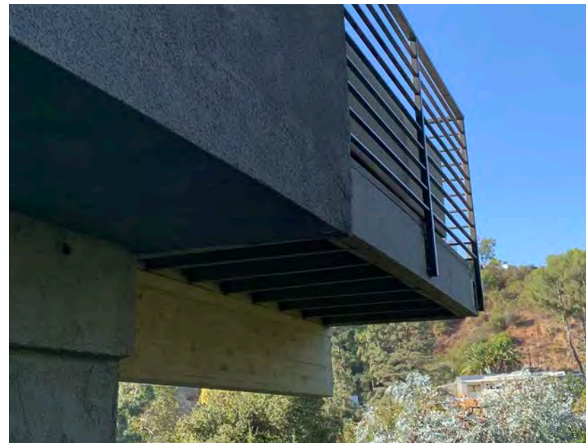
Partial view outside of the house and middle level deck and guard rail.
