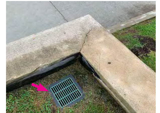
Iron Grate on the south end of the retaining wall
