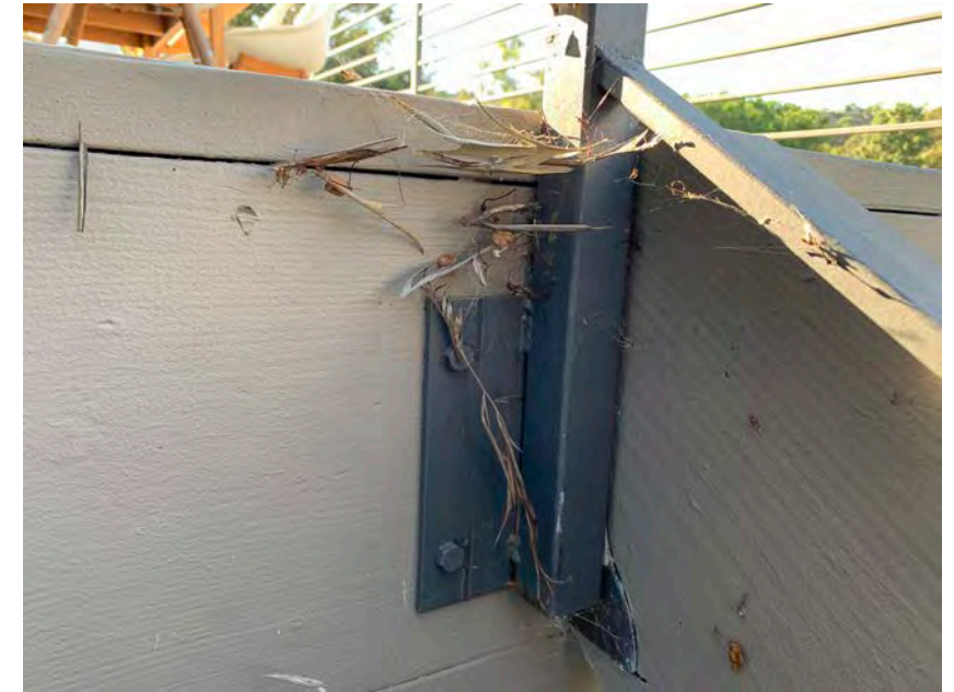
Connection of guard rail with the stairs and upper deck.
