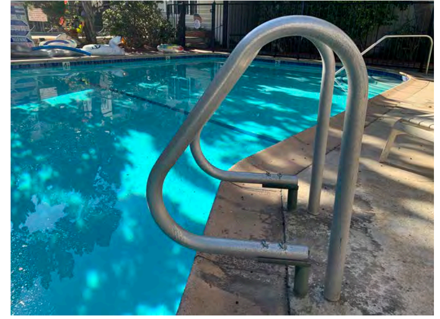
Railing of north in-wall ladder and concrete paving around the pool. In the back is the railing for the pool entry steps.
