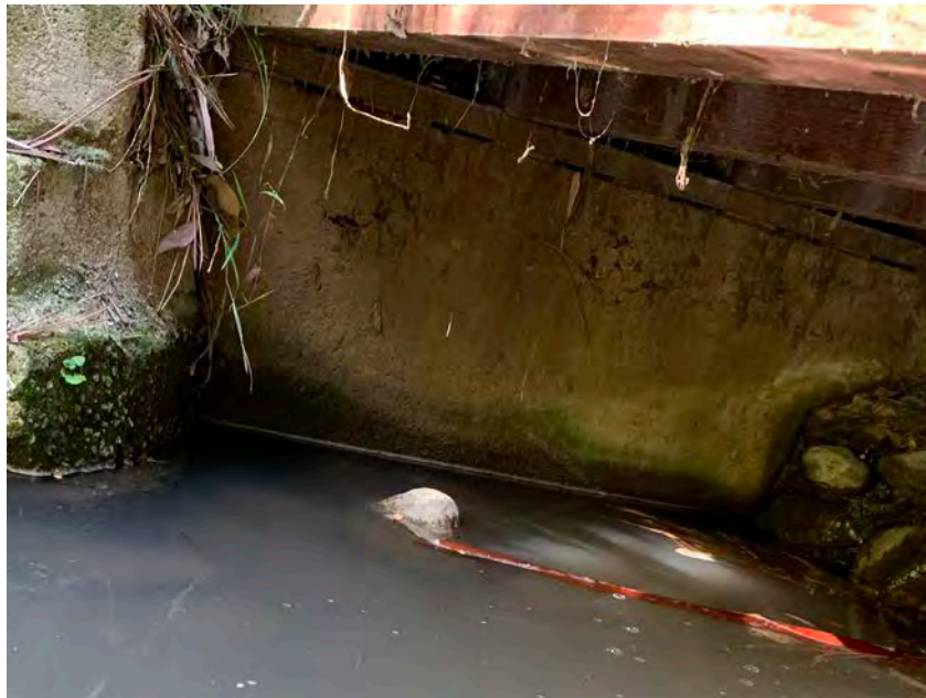
Under the bridge showing concrete base and beam on top where joists are attached.
