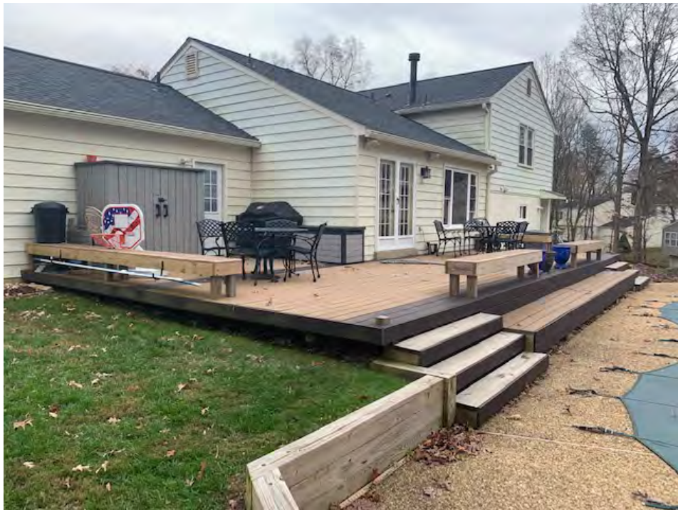
View of the deck and the back of the garage and the house, as seen from the northwest corner of the property. To the right is the pool showing only part of the pool cover.
