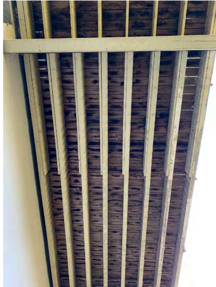
Closer look of middle level deck underneath.
