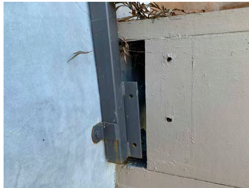
Connection of guard rail with the wall and upper. Piece of wood from the upper deck where guard rail was connected is missing.
