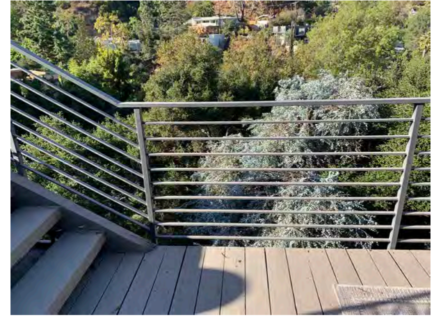
Guard rails, stairs and middle level deck.
