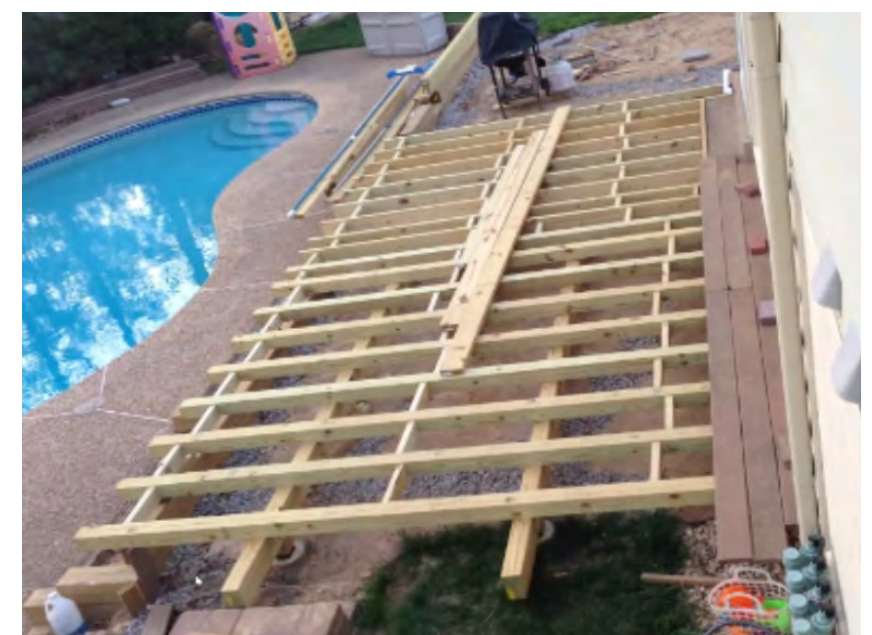
Showing part of the front and south side of the framing. Here joists rest on top of the beams. Also seen is the blocking.
