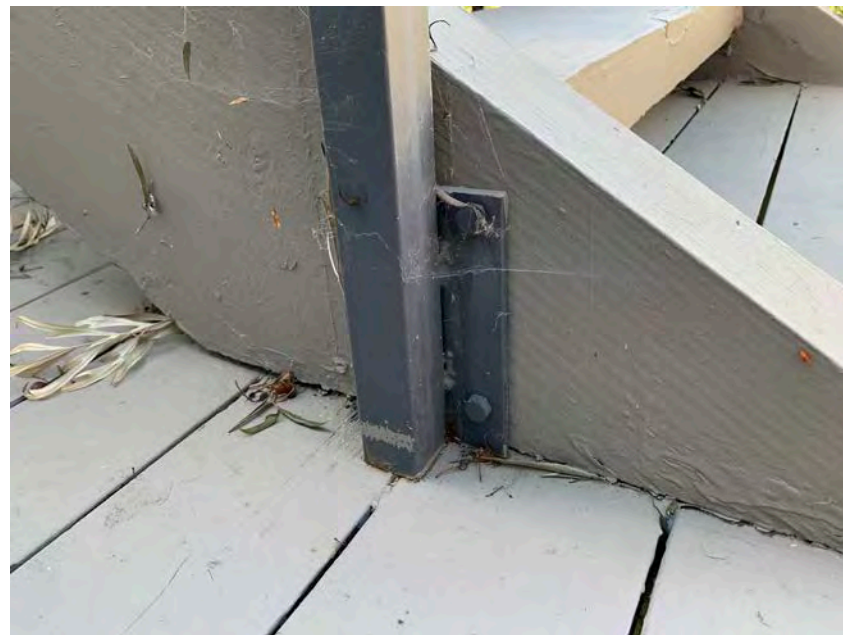
Connection of guard rail at the bottom of the stairs and middle level deck.
