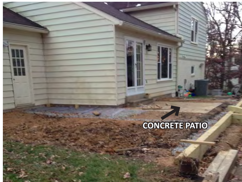
Photo was taking during grading part of the site at 2.5% sloping away from the house. There is a concrete patio that was not removed.
