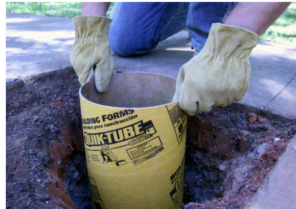
Concrete tube form used to pour in the cement for the footing.
