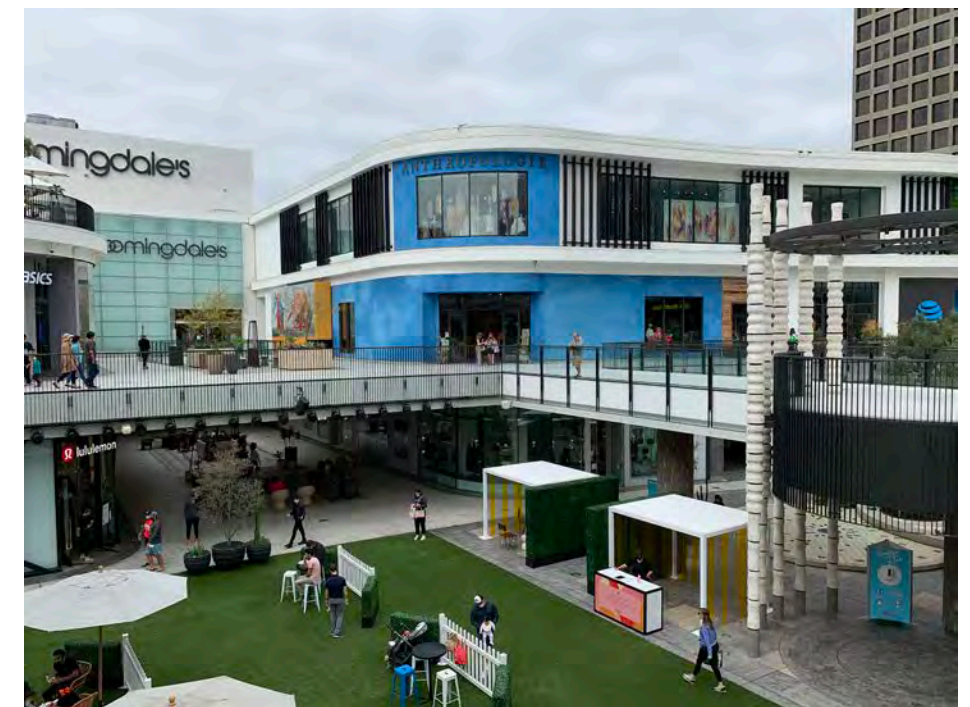
View of Levels 1 and 2.
