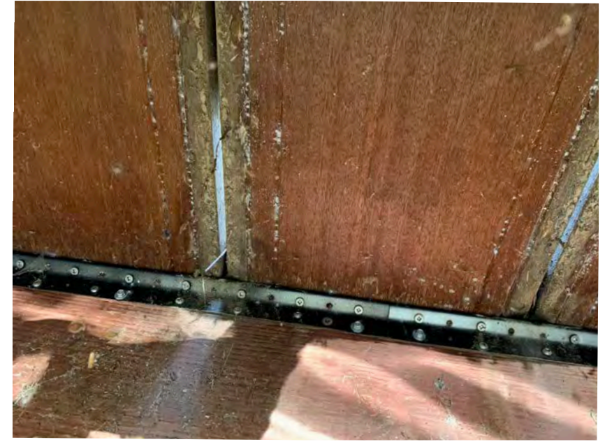
View under the decking (top) attached to the joist (bottom) with GRABBER DECKMASTER brackets and screws.
