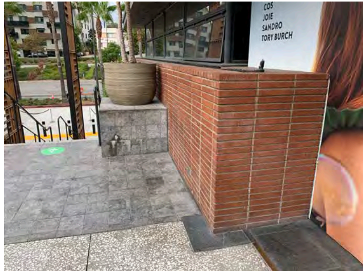
Planter with brickwork in stacked bond flatwork.
