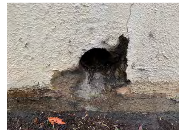
Close image of one of the drain holes
