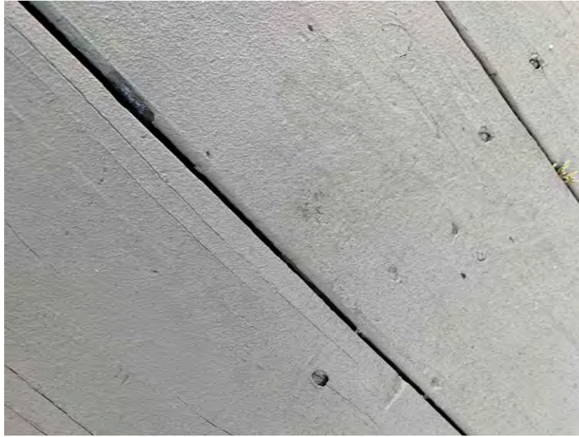
Spacing in decking and nails.
