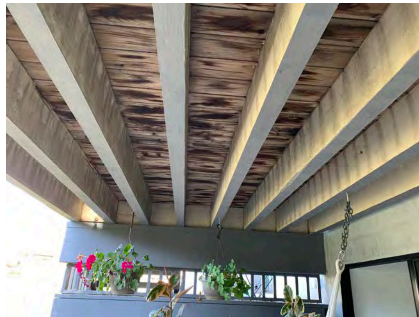
Ceiling of the overhead structure (upper level deck).
