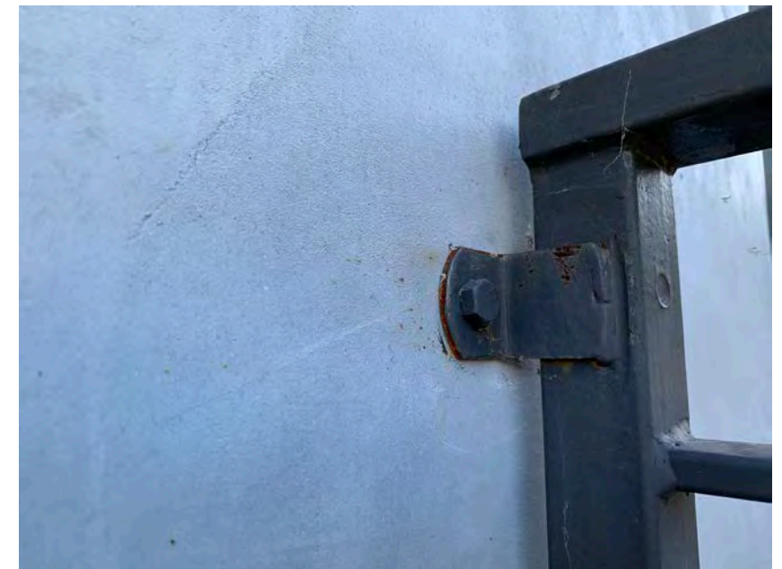
Connection of guard rail with the wall of the house.
