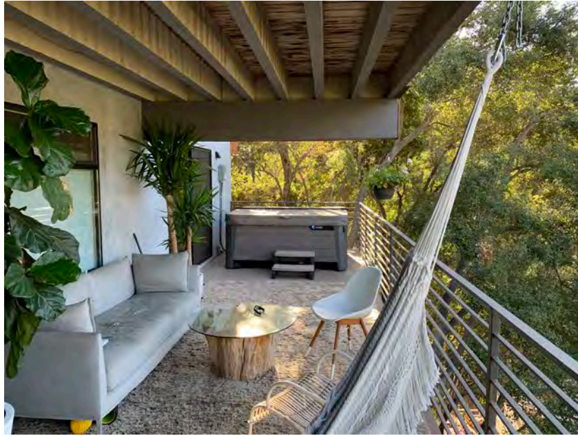
Ceiling of the overhead structure showing beam.
