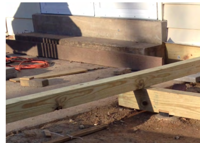
Existing step used to attach another ledger board. Used bottom step as the height of the decking. Also shown the concrete patio that was left and build the deck on top of it.
