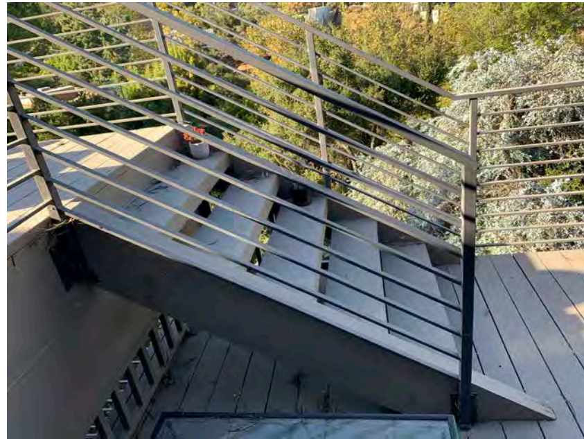
Stairs connecting the upper and middle decks
