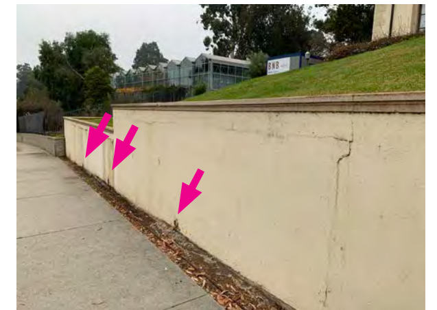
Drain holes along the south side of the retaining wall
