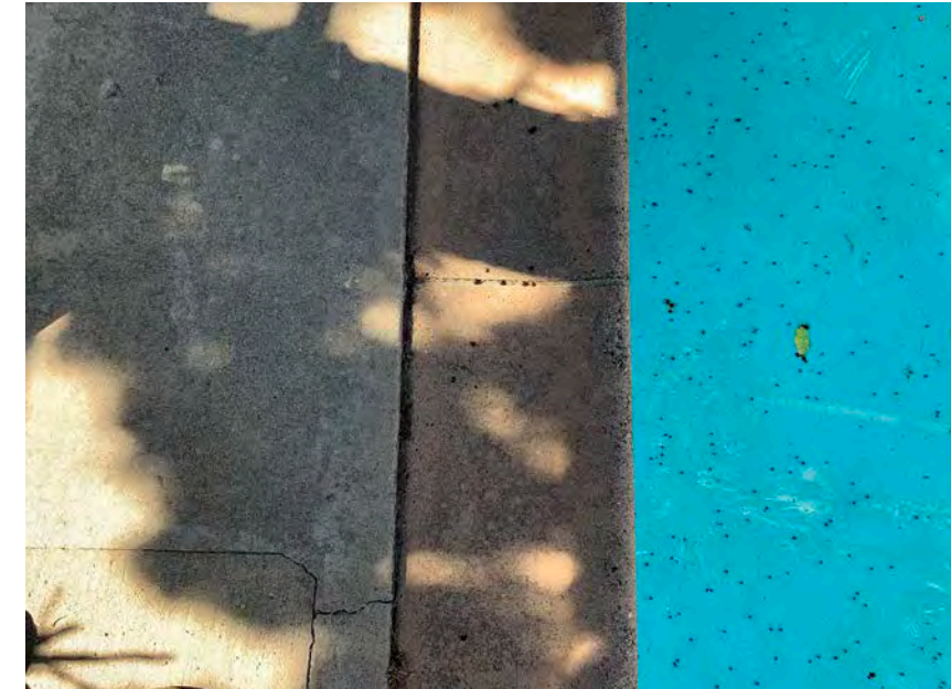
Top view of concrete paving, felt with sealant, paver pool coping and plaster.
