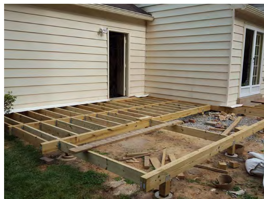
Framing in front of the garage, north side. The joists and beam are on the same plane. Joists look more like blocking.
