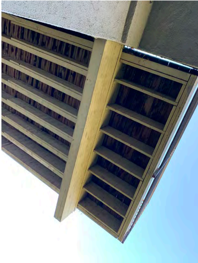
View of the middle level deck, joists, beam and part of the house.
