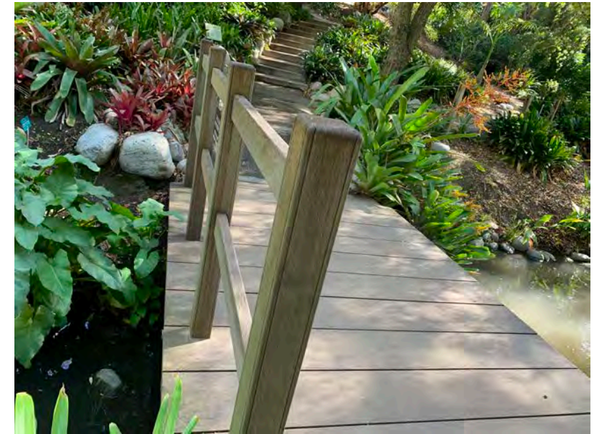
Looking at north side of bridge with guard rail.
