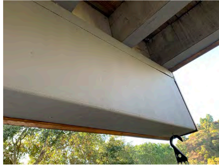
Close view of beam supporting overhead structure.
