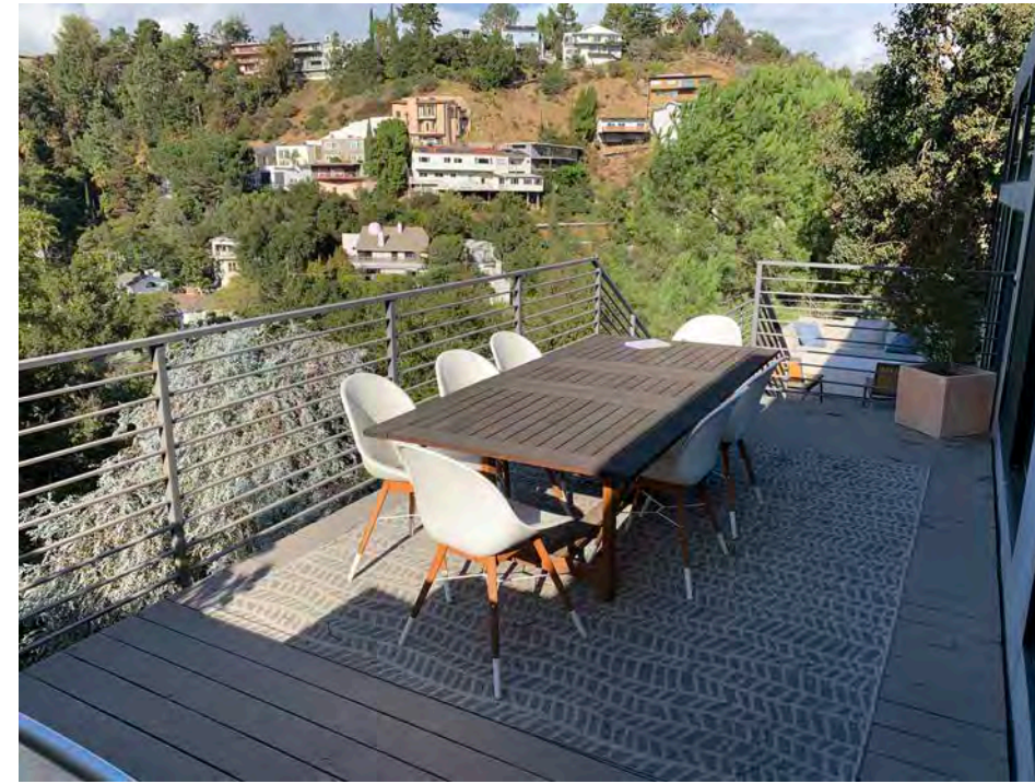
Upper level deck (overhead structure for lower level deck)
