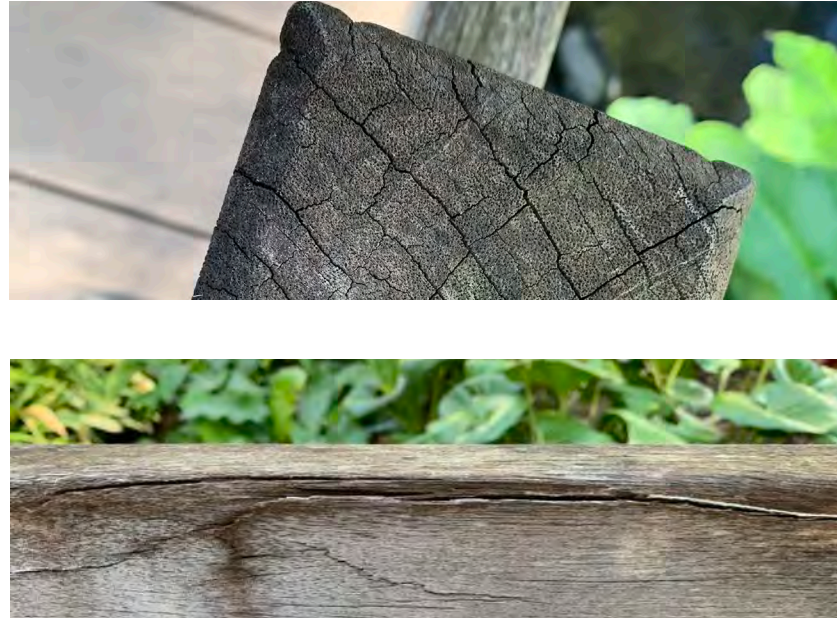
Guard rail post (top) and rail (bottom) showing cracks and water damage.
