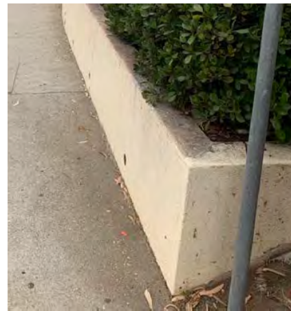
Front and north side of the wall
