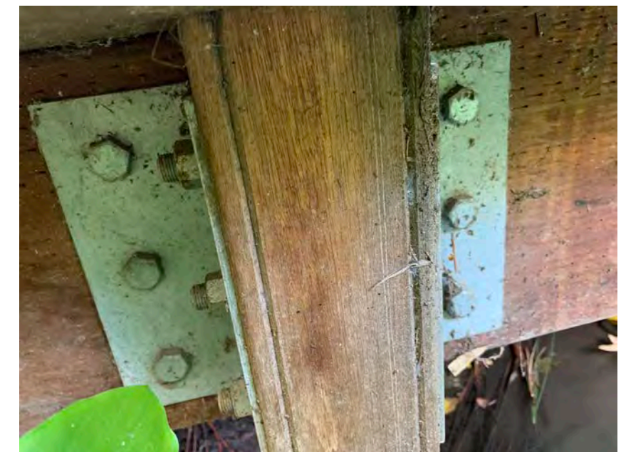
Close photo of bolts attaching guard rails and joists.
