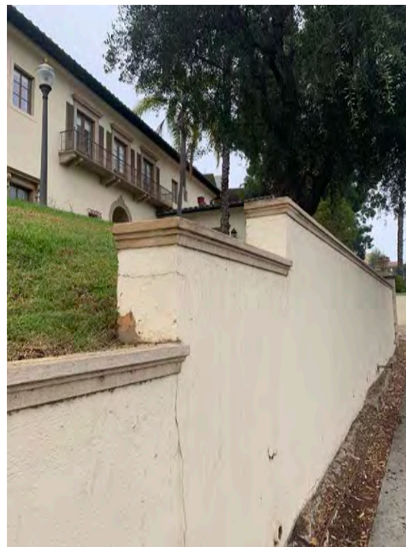
Front and south side of wall
