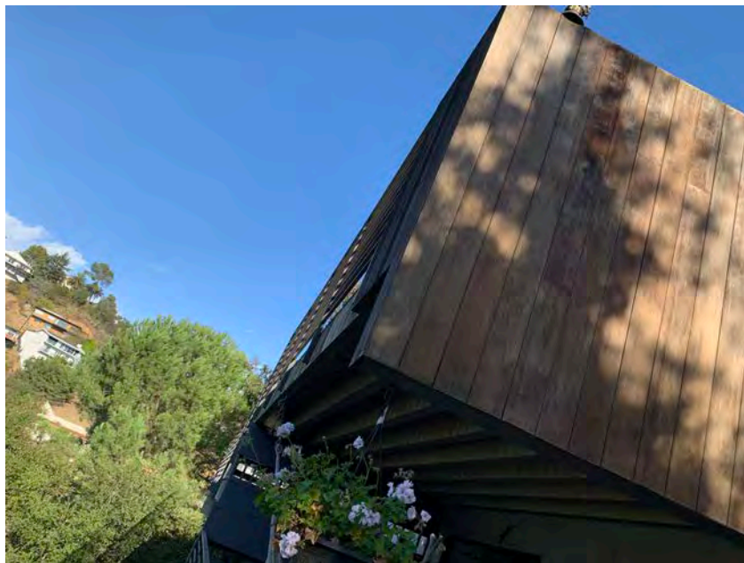
Overhead structure (upper level deck) and wooden guard rail.
